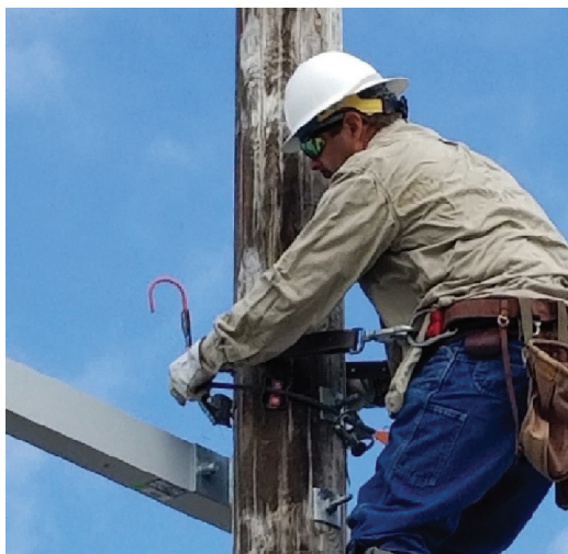
Foreman Tony Sienknecht completing pole climbing competency.
