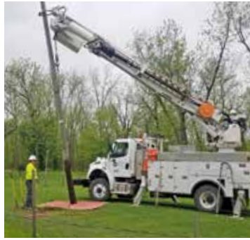
The GCREC line crew replaces a lift pole in a member's yard.
