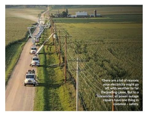
You might also see them replacing a downed utility pole, a painstaking process of removing the old and hauling in and raising the new, using trucks specifically designed for the job.
